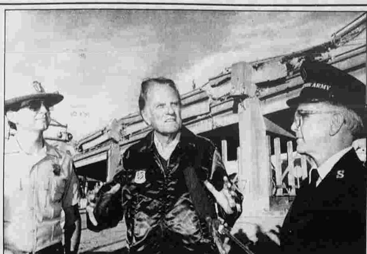
GRAHAM VISITS DISASTER SITE — Rev. Billy Graham, center, talks with California Highway Patrol Sgt. Bob Davis, left, and Salvation Army Lt. Col. David P. Riley at the crumpled Cypress structure of I-880 Monday. Graham offered a memorial service for rescue workers.
